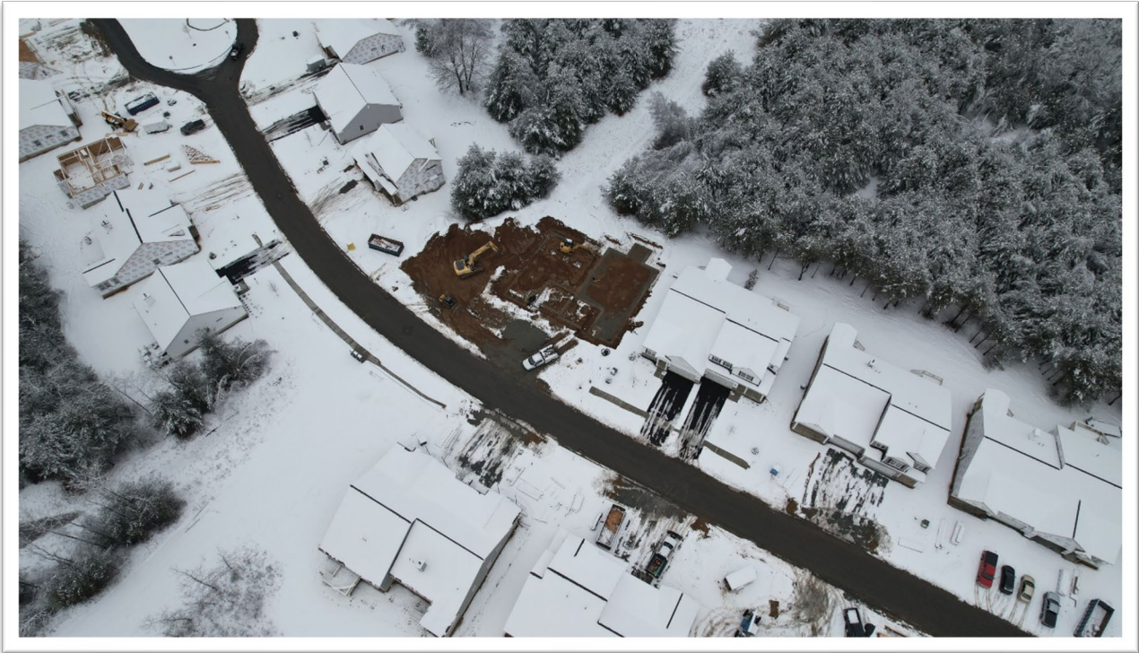
Figure 4. Residential homes under construction
