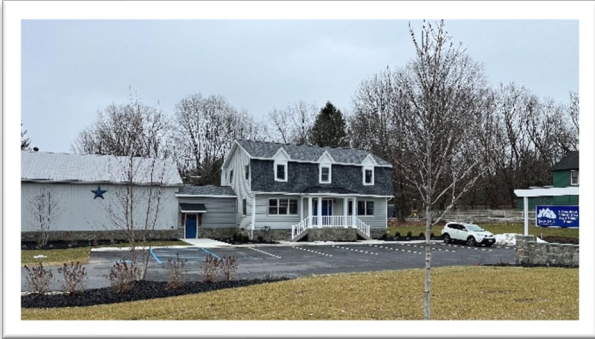
Figure 6. Saratoga Construction, Approved 2021
