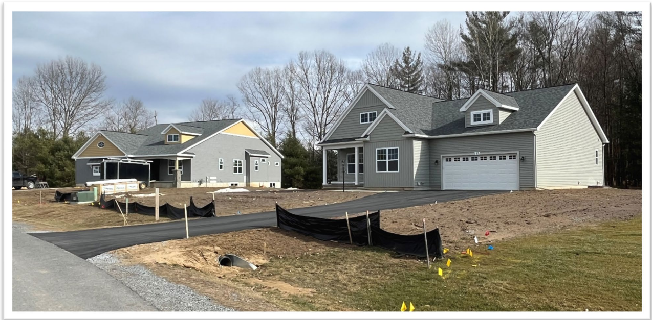
Figure 4. Residential homes under construction
