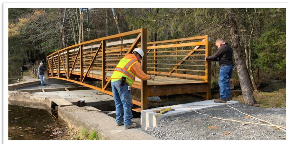
Figure 2. Pedestrian Bridge Installation at Camp Saratoga
