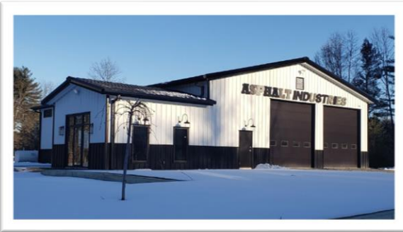
Figure 6. Stanley Business Facility, Approved 2020
