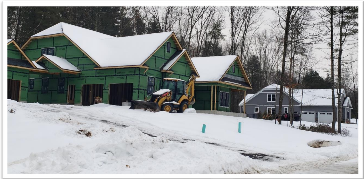
Figure 3. Residential home under construction
