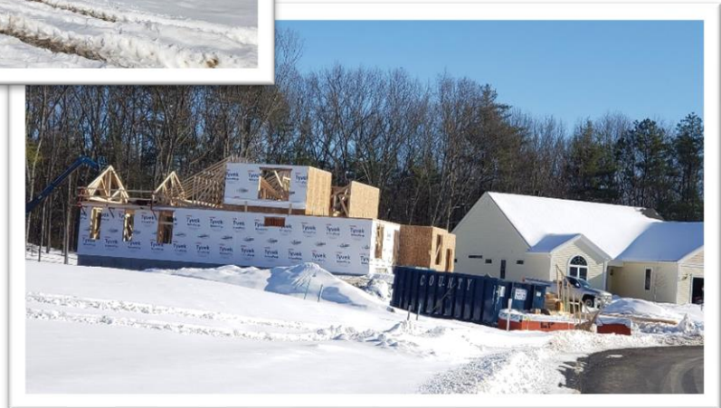
Figure 10. Residential homes under construction
