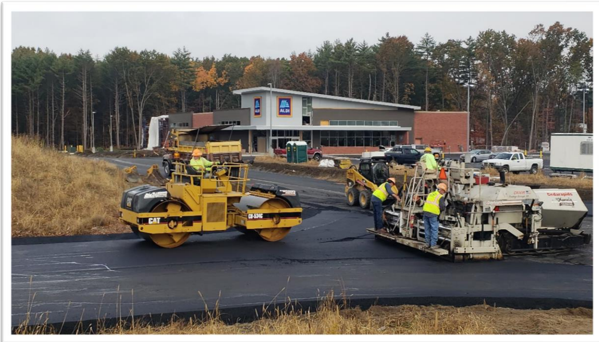
Figure 7. ALDI at Wilton Marketplace and the construction of Marketplace Road
