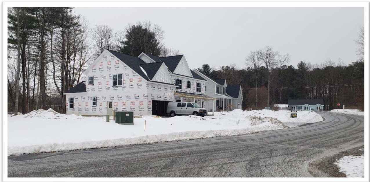
Figure 1. Residential home under construction
