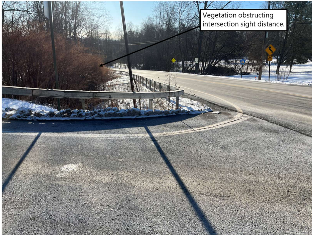
Photograph 5: Looking left (D.L) from Gailor Road westbound at Parkhurst Road
