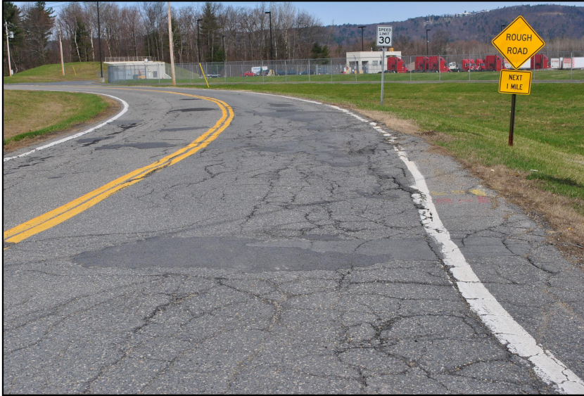
Deteriorating pavement along North Road
