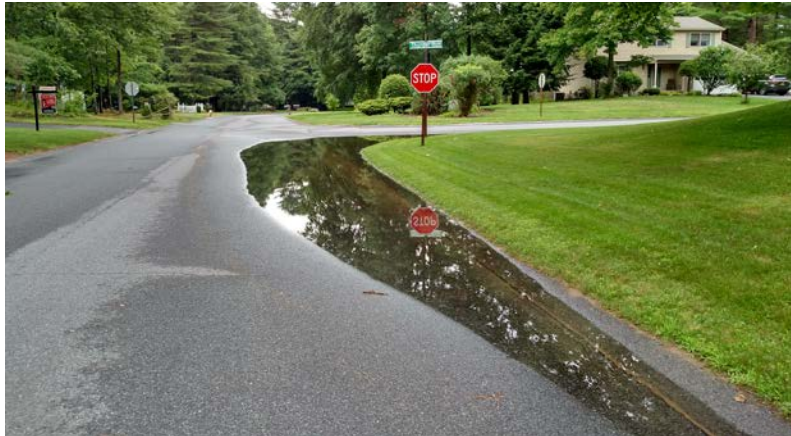
Figure 19: Water Unable to Drain off Pavement Surface
