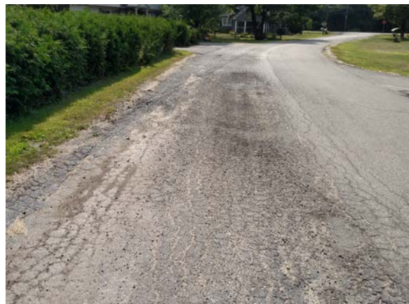
Figure 18: Raveling of Asphalt Surface
