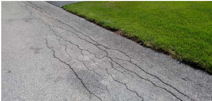
Figure 12: Edge Cracking
