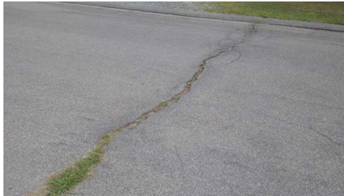
Figure 10: Transverse Cracking
