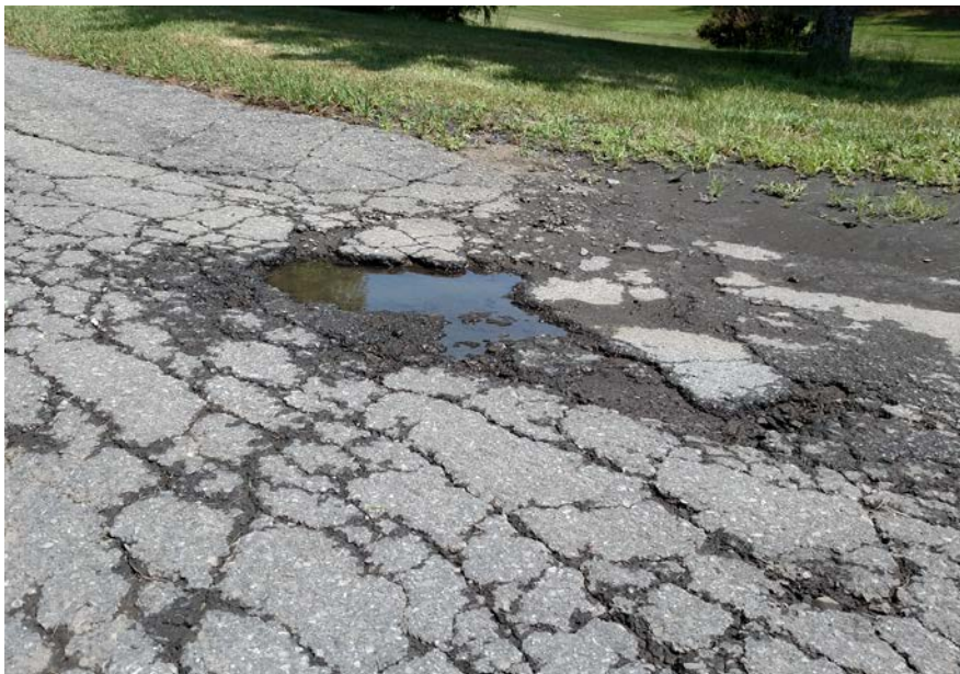
Figure 14: Pothole Resulting from Alligator Cracking
