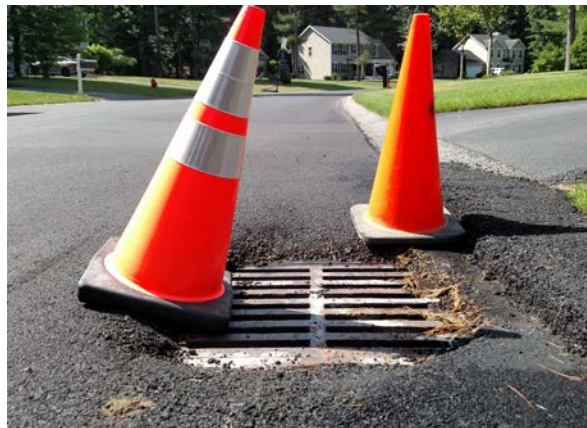
Figure 20: Structure Uneven with Pavement Surface
