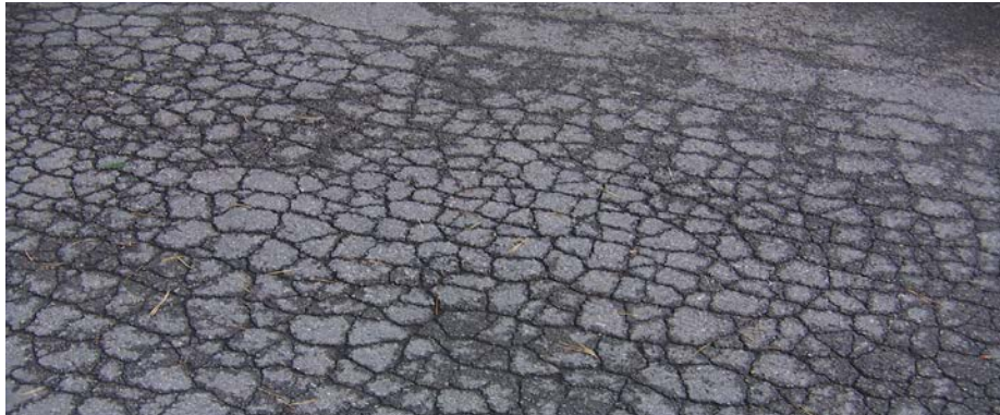
Figure 11: Alligator Cracking
