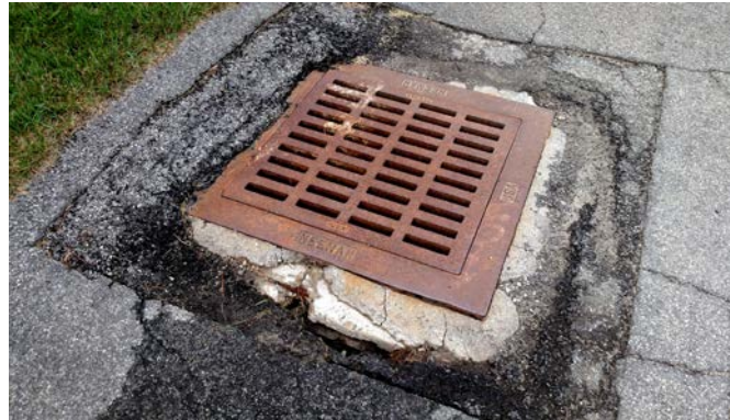
Figure 13: Deteriorating Patch Around Structure
