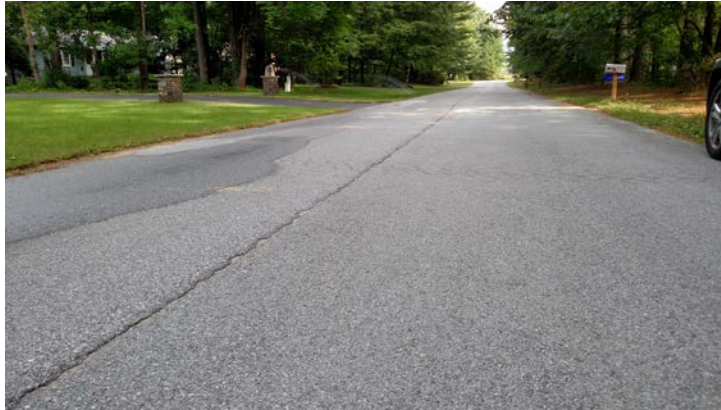
Figure 9: Longitudinal Cracking
